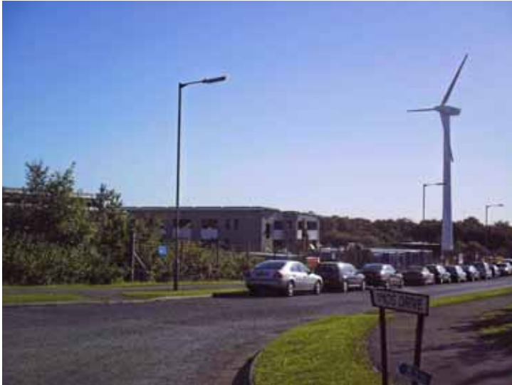
Figure 8 A second-hand Vestas 225 at the Green House, Annfield Plain, County Durham. North Energy carried out the initial feasibility study for this building
